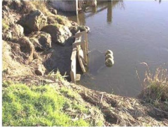
Figure 28. Self-regulating tide gate
